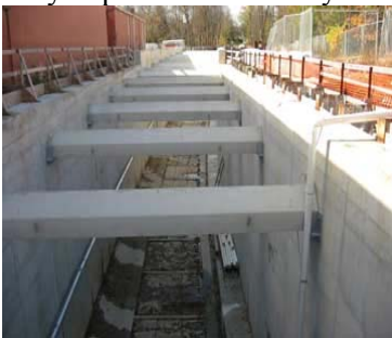
Early work on Hingham Tunnel (RJA)
